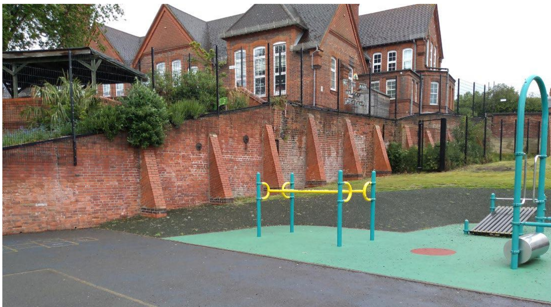
South-facing elevation showing modern buttresses
