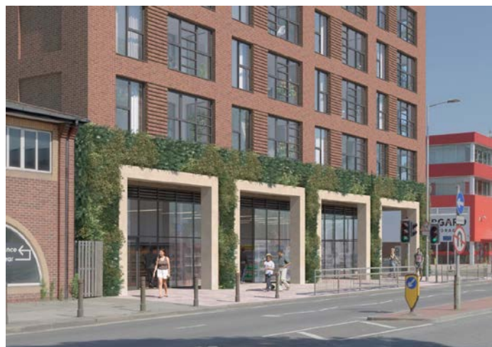
Fig. 6 - Colonnade looking northwest across Caversham Road
